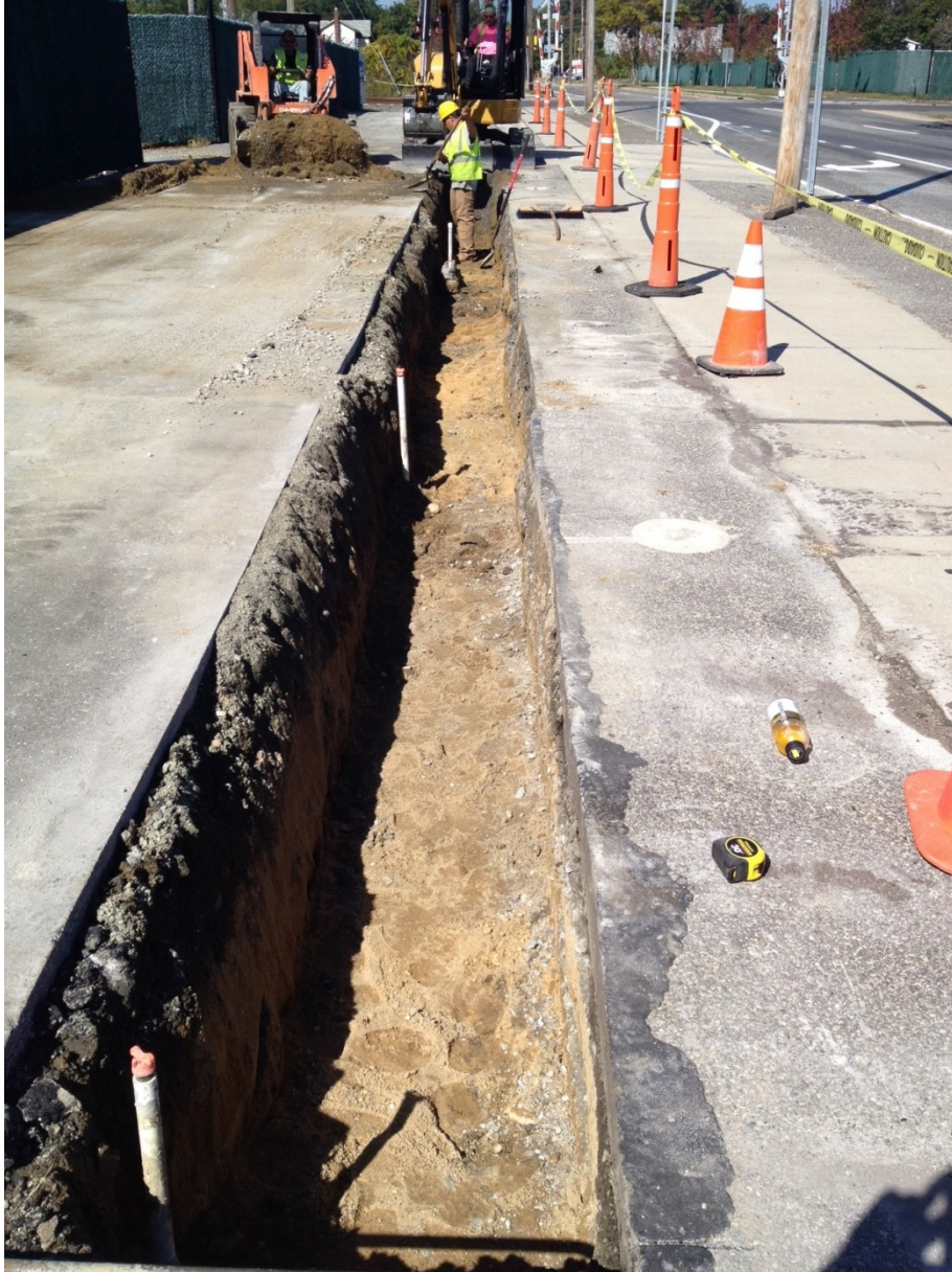
Excavated trench at 60/66 North Clinton Avenue adjacent to Clinton Avenue
