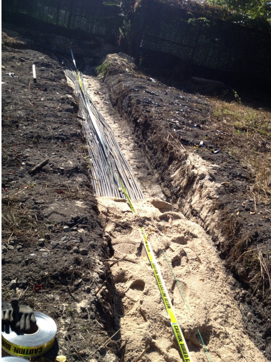
Oxygen supply lines and backfilling at 60/66 North Clinton Avenue
